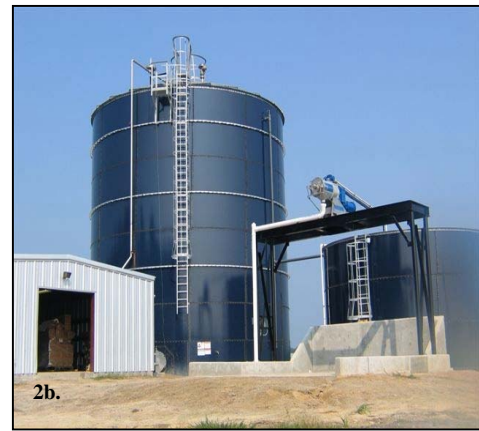
Figures 2a and b. Aerial view of BR Harris Farm and image of fixed – film mesophilic digester with settling tank and fan separator.
